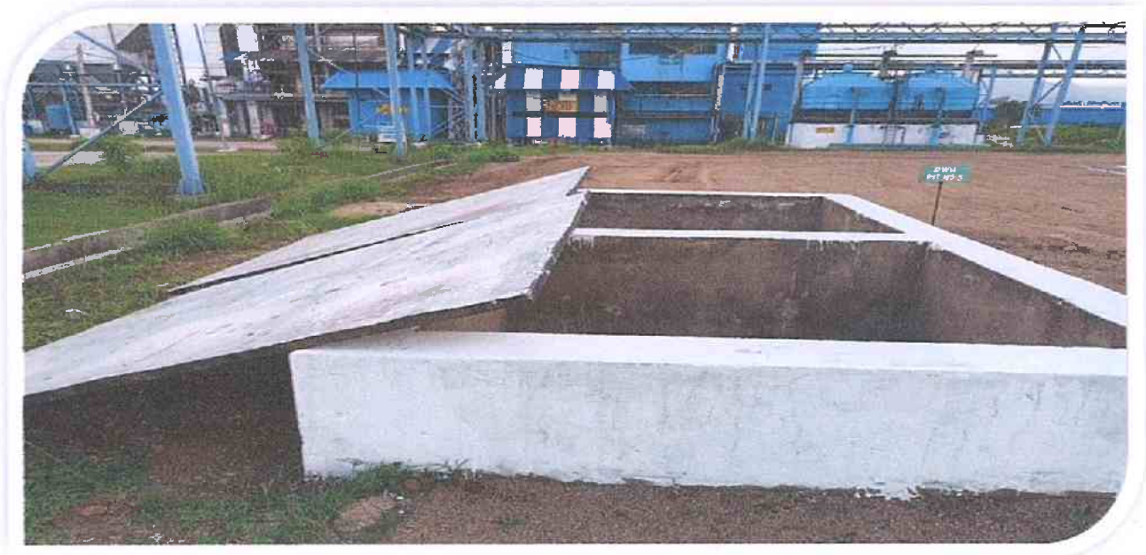
Annexure-V: Photos of Rain Water Harvesting Pit
